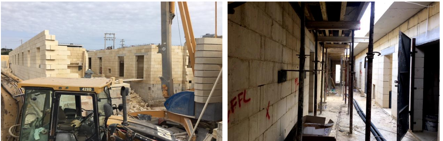
Figure 17: Works on site at CORRS, Mtahleb
