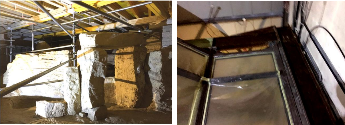
Figure 15: works at the Hal Saflieni Hypogeum
