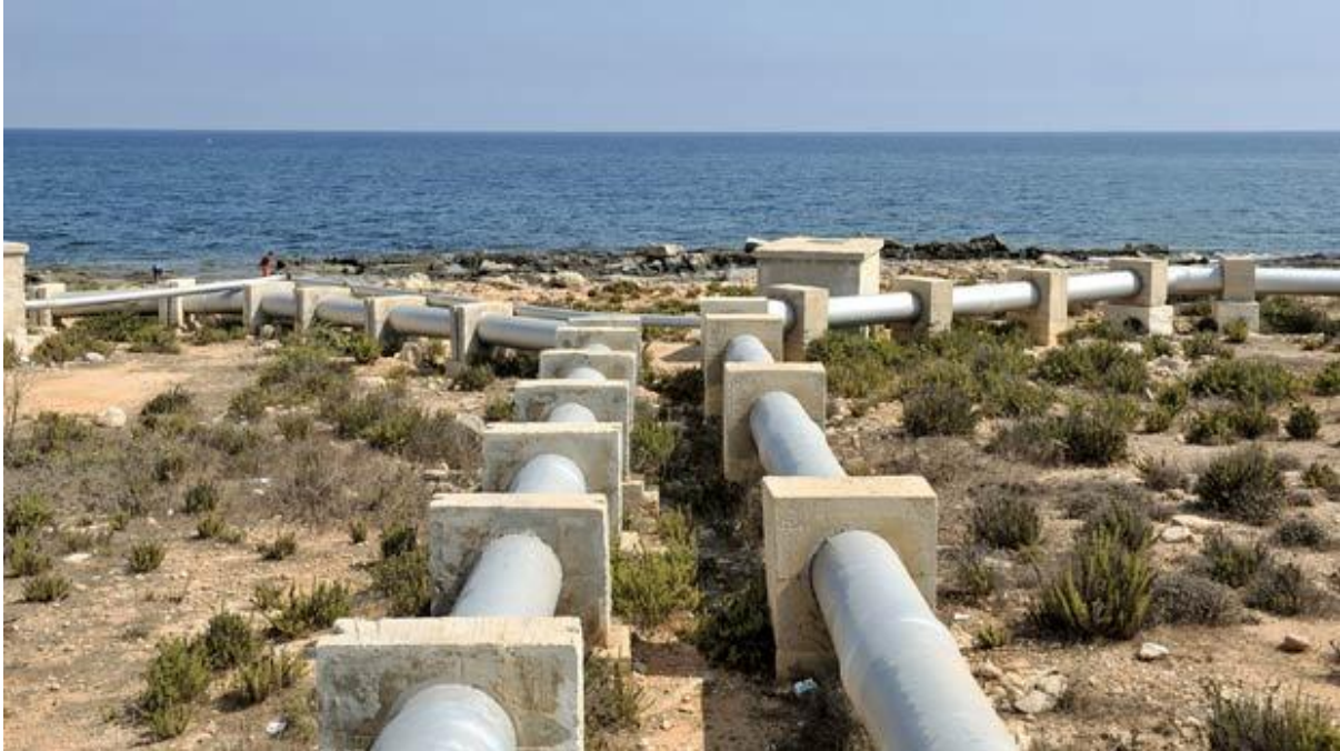
Figure 3: Reverse Osmosis Plant in Malta
