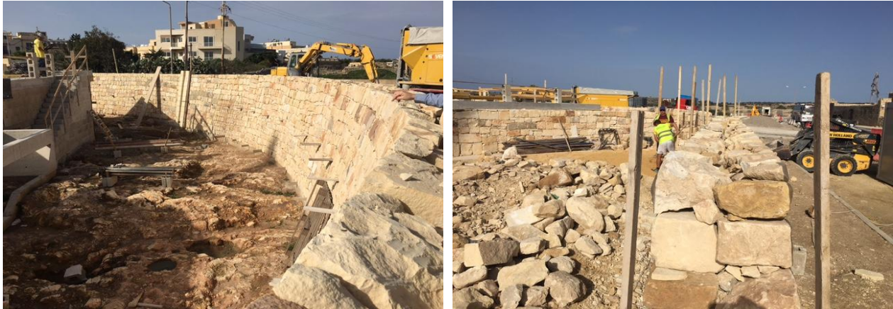
Figure 13: Works on site, Project MT02/7
