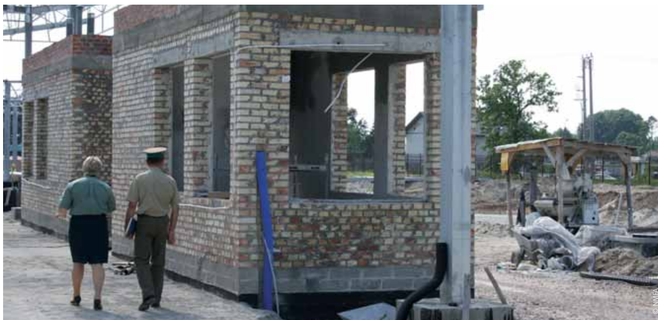
The modernisation of the Terespol border crossing at the Polish-Belarusian border at the edge of the Schengen area was one of the largest projects supported by the Norway Grants.
