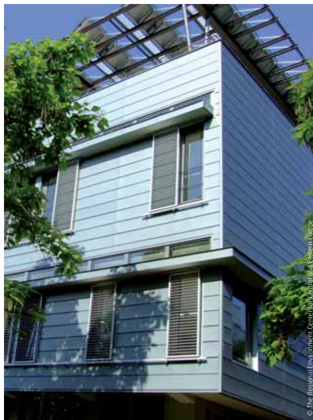
In Hungary, the Regional Environment Centre has been made into a zero-emissions conference centre.
