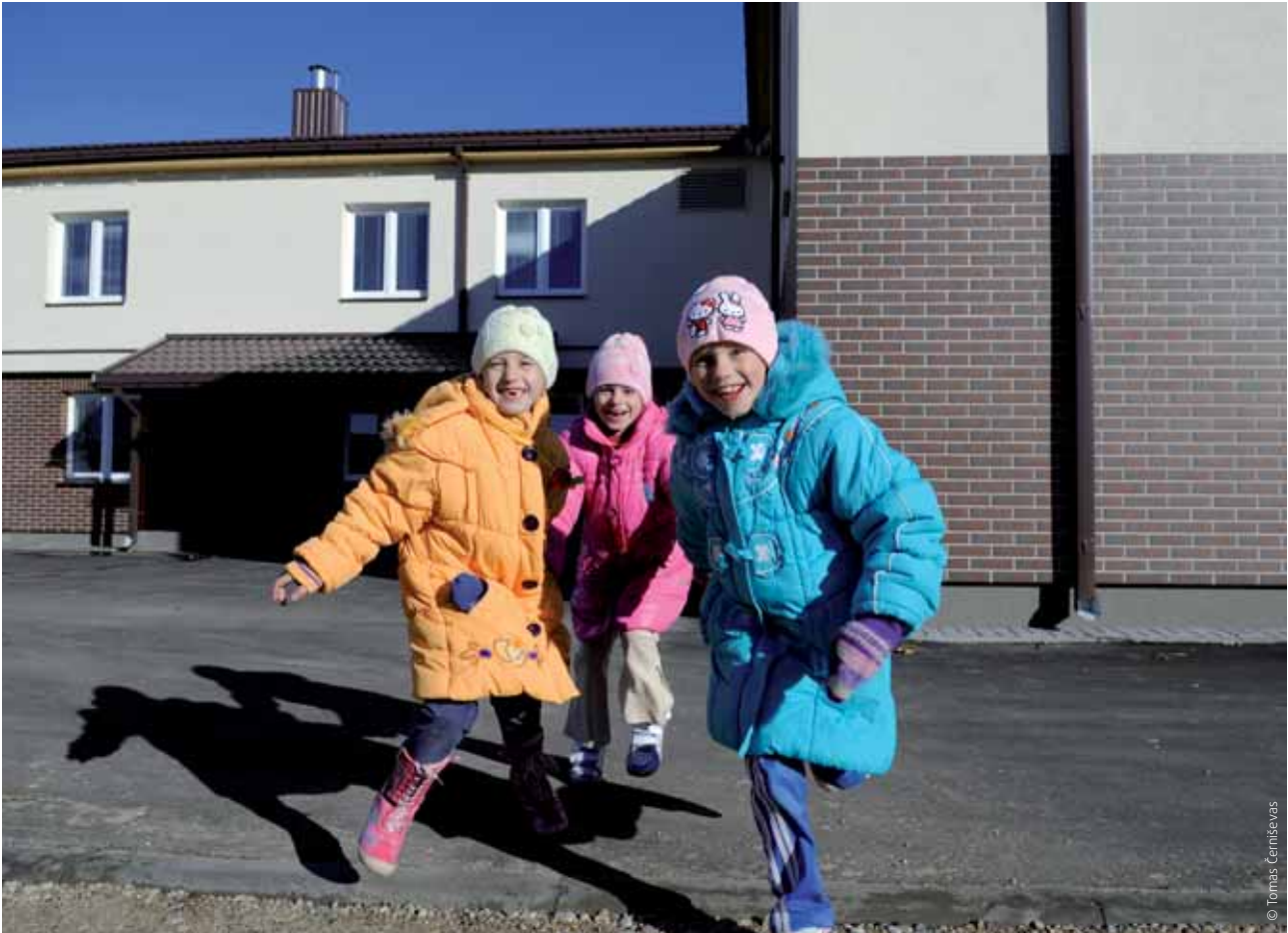
Renovation of the foster care home in Beizionys in Lithuania has helped to improve living conditions for children.
