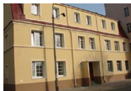
350 public buildings in Poland will be insulated and made energy efficient, a number of them with renewable energy sources.
